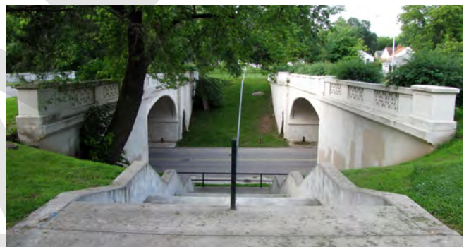
FIGURE 4.7 EXISTING GATEWAY/UNDERPASS BELOW THE PASEO
