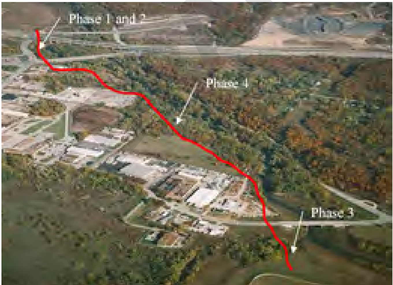
FIGURE 6.10 DODSON INDUSTRIAL DISTRICT FLOOD WALL LEVEE
