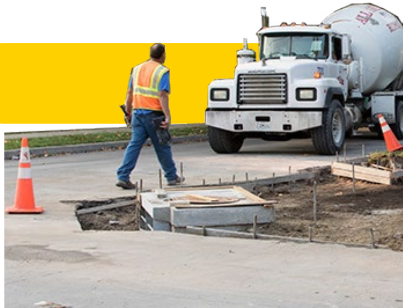
GO KC Programs aims to repair and replace sidewalks citywide. IMAGE CREDIT: KCMO
