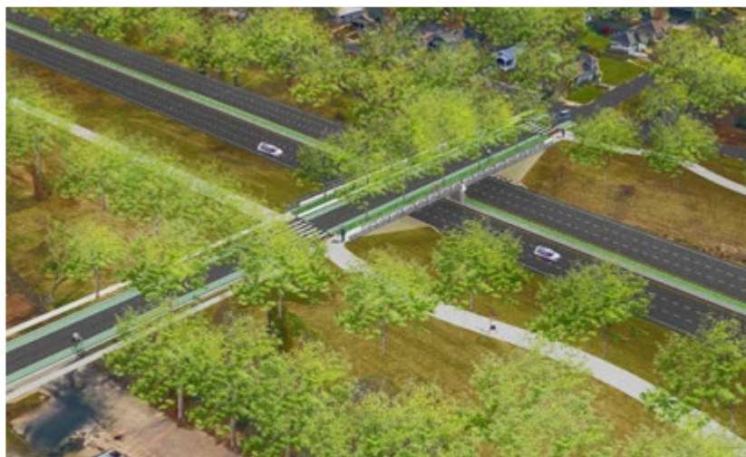
TOP High visibility color painted bike lane along Highway 71 will provide better connections and access to other destinations within the Swope Area. BOTTOM View of bridge with bike lanes.
