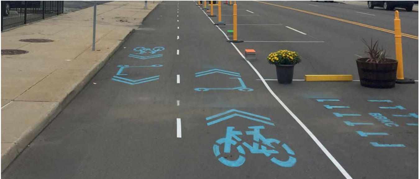
BETTER BLOCK KC OAK STREET DEMONSTRATION PROJECT, OCTOBER 2018
